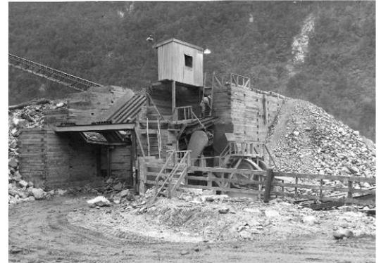
During the building of the second tunnel spoil was brought out of the tunnel on a conveyor belt and across the tailrace to a dumping point on this embankment, from where it was spread using dump trucks.
